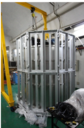
(e) Install the lead brick shielding.
