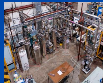
Liquid Argon Test stands at Proton Assembly Building
